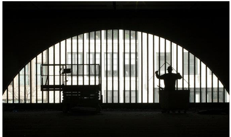
The Boston Public Library’s major renovation project is underway at its Johnson building.
