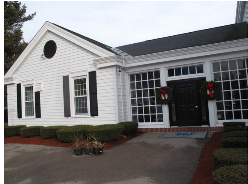
Main Entrance, Police Station
