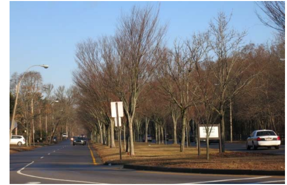
Traffic on the Blue Hills Parkway has increased by over 5% per year from 2009 to 2012.
