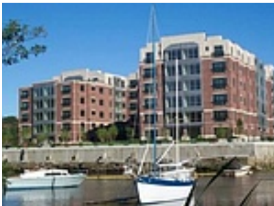
88 Wharf Street Apartments
