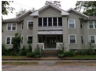
Condominium Units at 17 – 19 Revere Street
